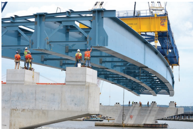
The project's first steel girder assembly is slowly lowered to its final location atop a pair of concrete piers.
