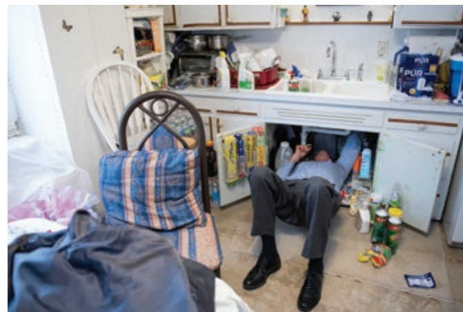
Edwards gets under the sink to check Elnora Carthan's plumbing.
