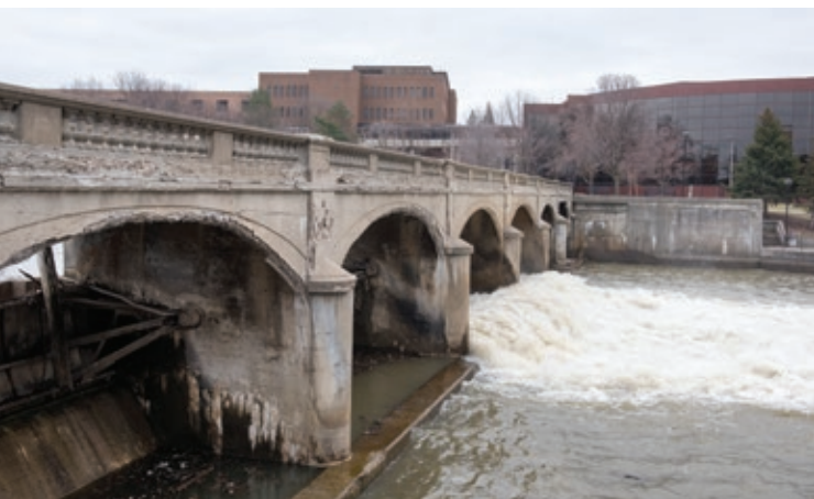
A spillway along the Flint River.
